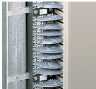
Installation example: Matrix patchboards in a frame
