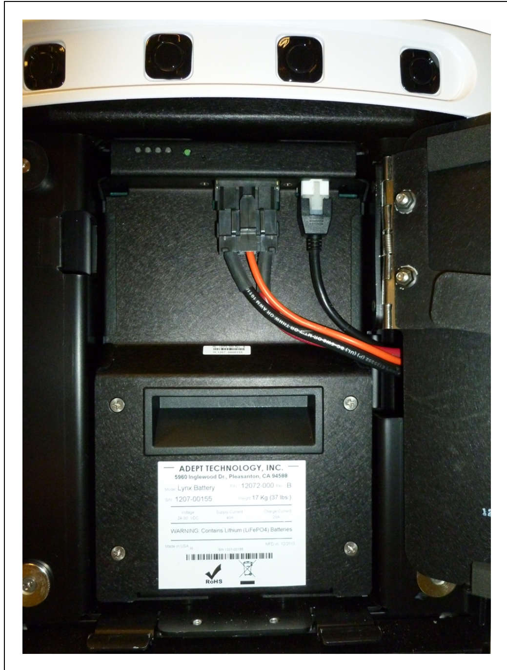
Figure 8-6. Battery Compartment, Connectors
