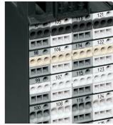
Insulation stop is in place.
