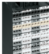
Insulation stop is in place.
