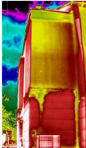
What a thermal imaging camera sees
